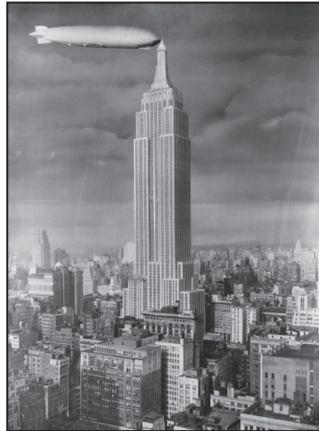
A simulated image of a dirigible docking at the mooring mast
