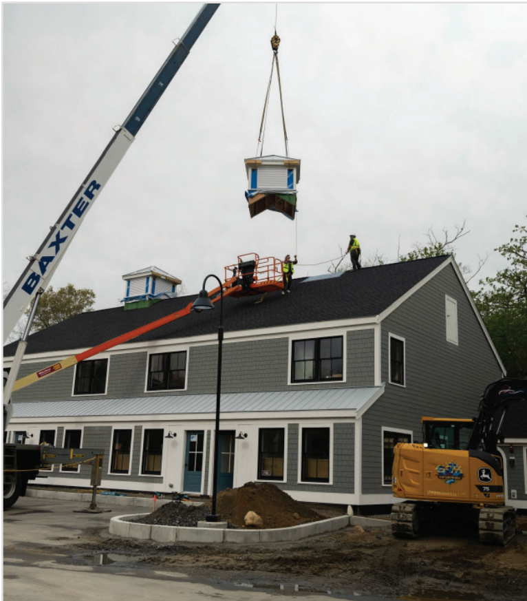
Figure 7: An Affordable Housing Development Under Construction in Orleans, One of the First Built in the Town’s Form-Based Downtown Housing Overlay District 22
