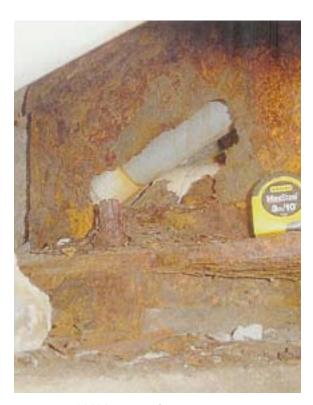
Figure 5: 100% section loss to stringer (Source: DCR 2006 Inspection Report)
