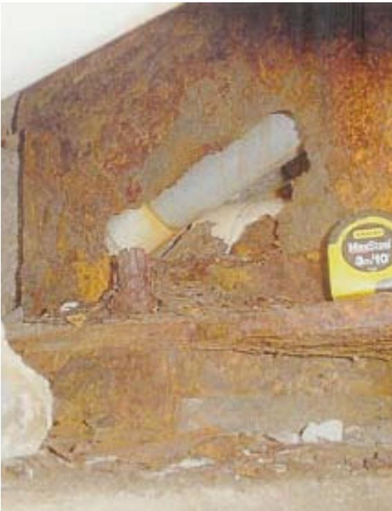
*Figure 5: 100% section loss to stringer
