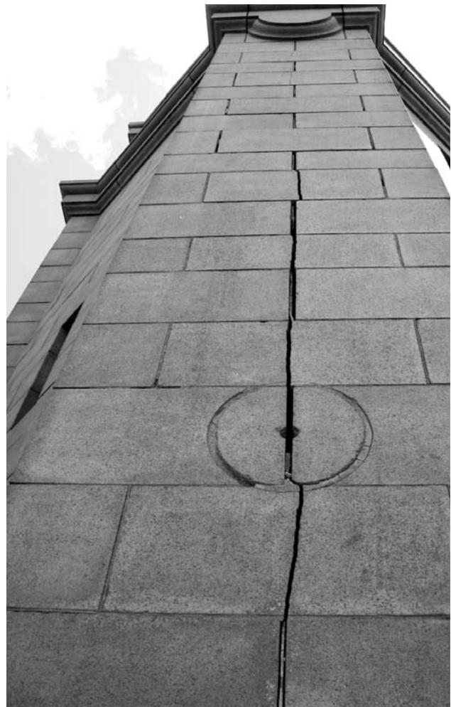
*Figure 8: Cracking in Pier
