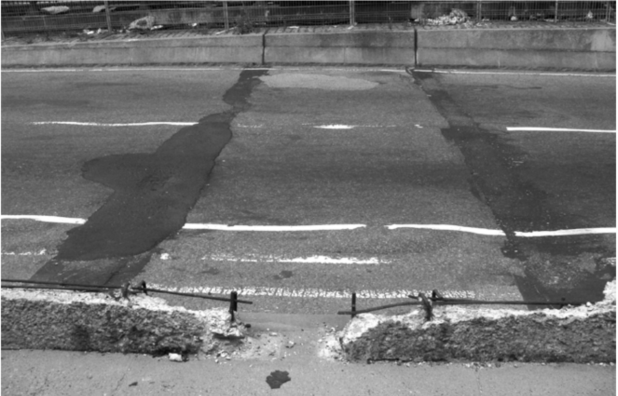
Figure 3: Longfellow Bridge Deck (Photo by Peter Begley)
