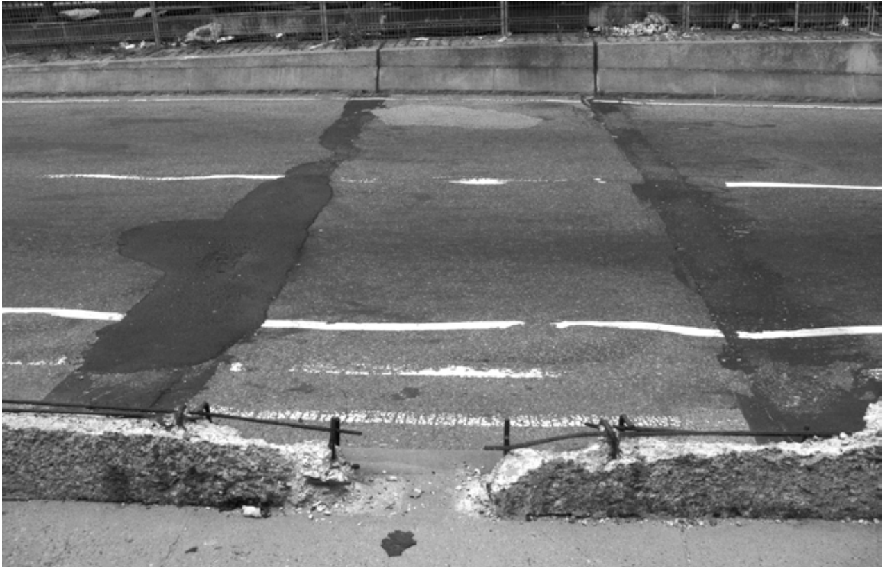
Figure 3: Longfellow Bridge Deck (Photo by Peter Begley)
