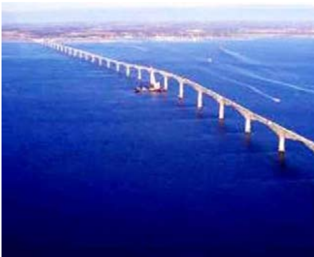
Figure 9: Northumberland Bridge Nearing Completion (1997)
